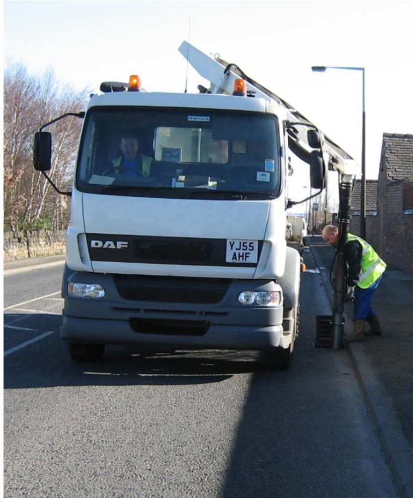
'Wet Spot' team at work with one of the new gully cleansing machines
