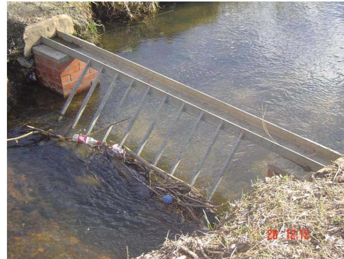
Wyke Beck trash screen (above) and Fearnville cut-off drain (below)
