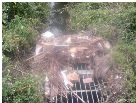
Cock Beck grid at Stanks (4 Sep 06) before (left) and after (right) fortnightly clearance
