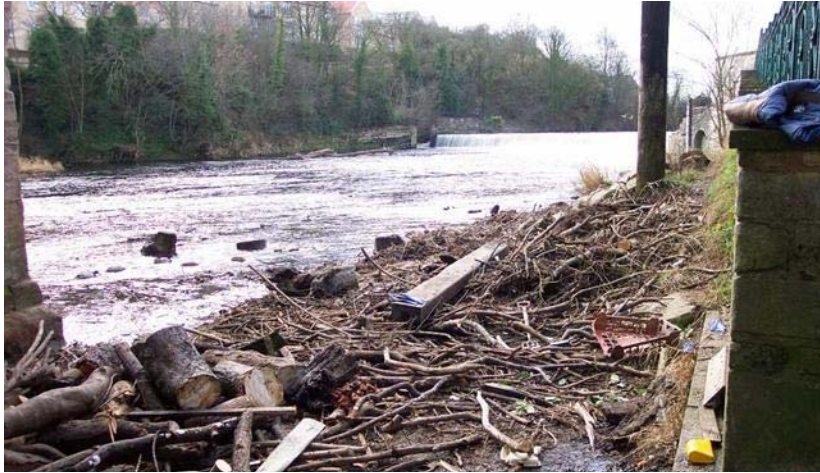
Tree trunks removed from under bridge on the River Wharfe at Wetherby (sawn into sections ready for removal)
