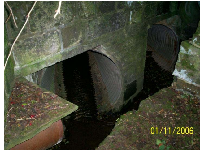
Entrance (above) and exit (below) to Carlton-Bramhope highway culvert.
