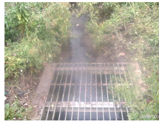
Cock Beck grid at Stanks (4 Sep 06) before (left) and after (right) fortnightly clearance
